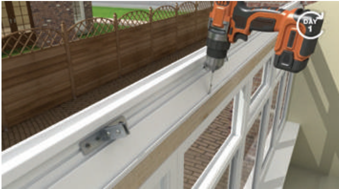
Timber packer and structural ringbeam are sealed and secured to the top of the window frames.
